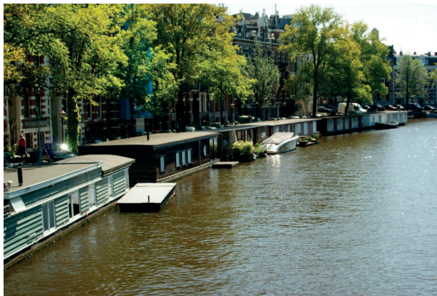
Figure 1. An example of floating residential structure in Amsterdam
